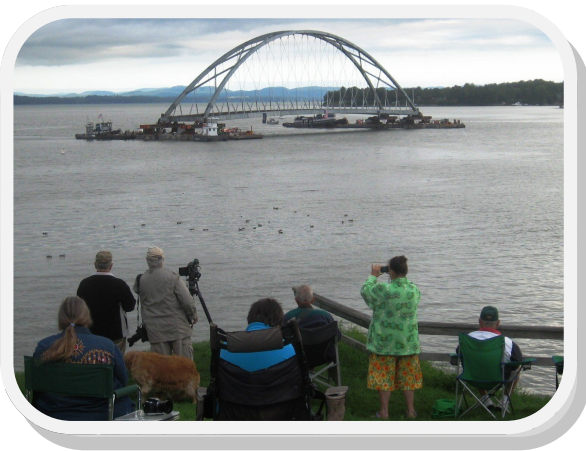
Above, the center span completed and making it's way on barges to be joined with the bridge
